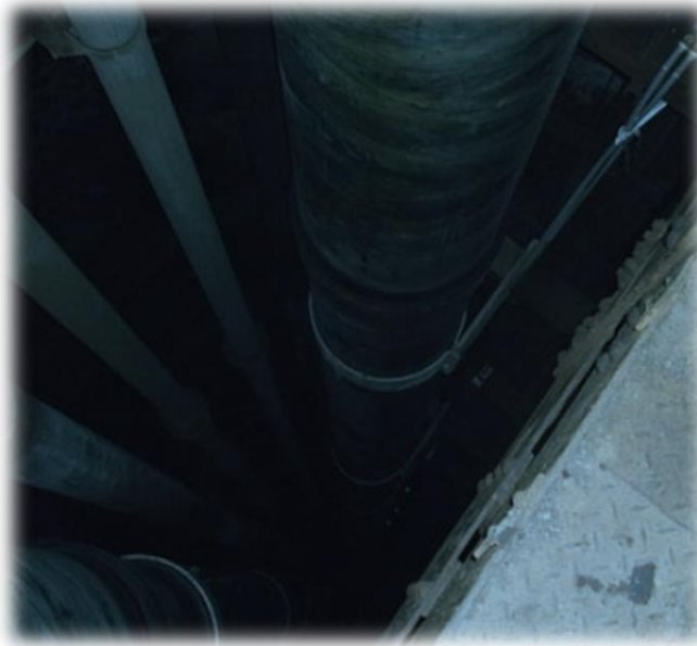
Cladding pipes in a shaft before shaft filling
